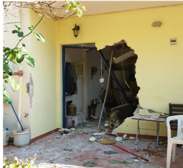
Figure 3. Damage from the falling rock on the impacted house in Ponti, Lefkada, Greece.
